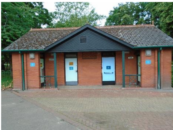
East Park Road - Spinney Hills Ward
